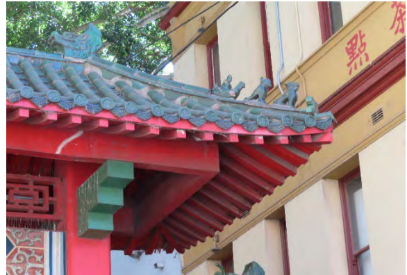
Figure 4.40 Symbolic ceramic features on the roof at the eastern bay of the south elevation.
