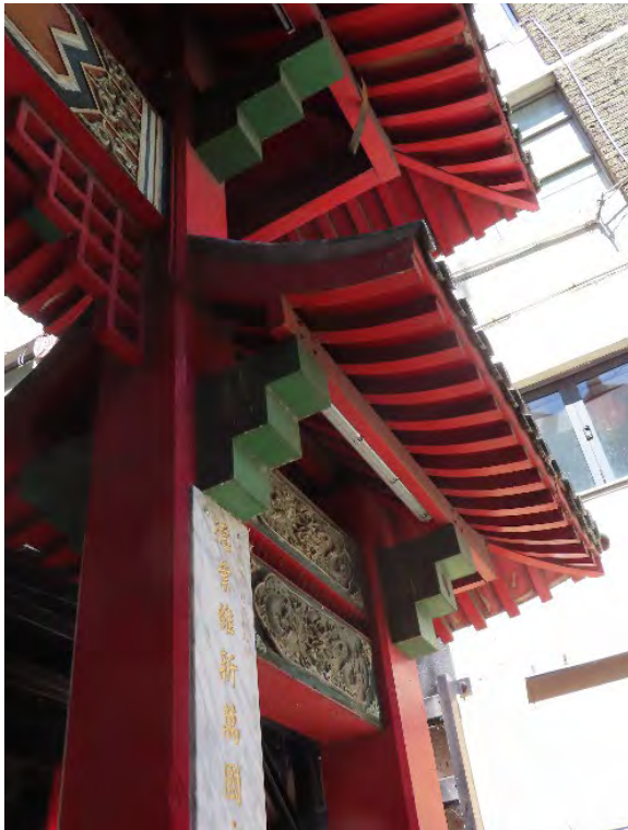
Figure 4.6 Underside of the curved timber rafters and stepped brackets of the west gateway, showing the lower and upper roof of the north elevation.
