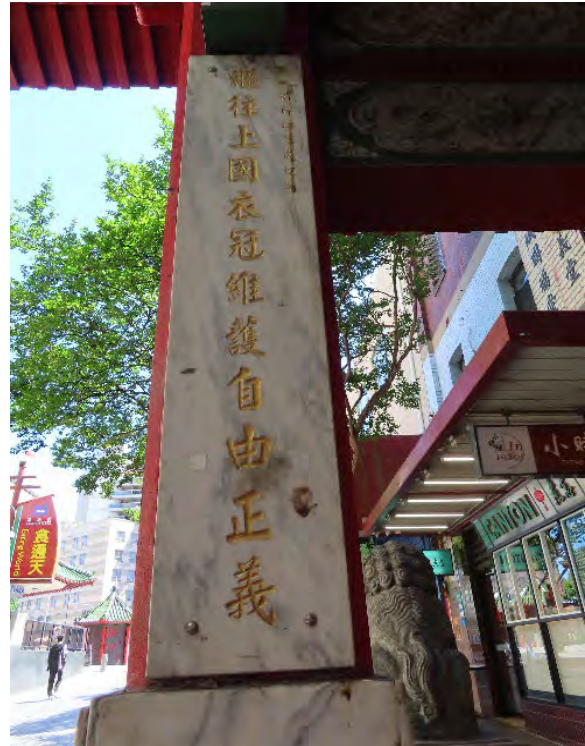
Figure 4.13 Gateway plaques on the column of the western bay.
